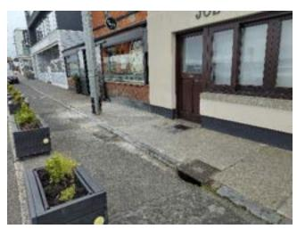
Wherever gutter downpipes discharge at surface level (as shown here, R and below) rather than into sunken gullies, there is a very cost-effective opportunity to incorporate shallow rain garden into the street design.
