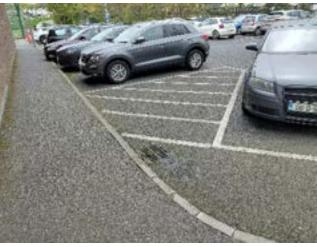
Even a narrow area along a hedge can be sunk down to create storage for stormwater (R).
