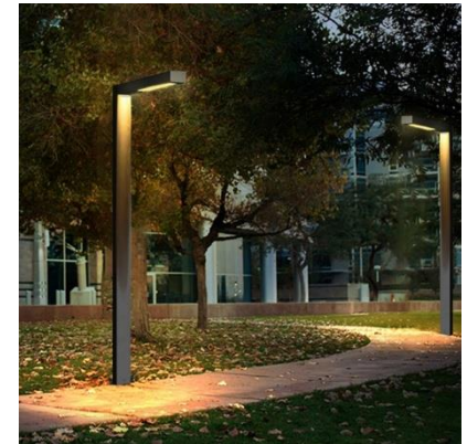
Figure 11-27: Example of full cut off residential lighting
